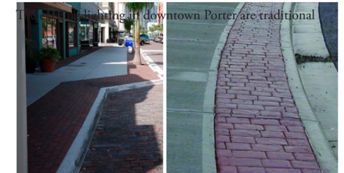
Photo 3-4. Brick paver band. Photo 3-5. Stamped Concrete band.
